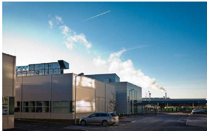
AAC new facilities at TFZ in Wiener Neustadt (Left: hall and labs with offices)
