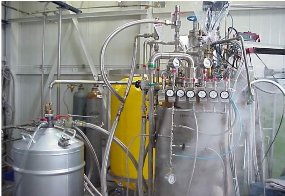
Slush production plant (laboratory)
